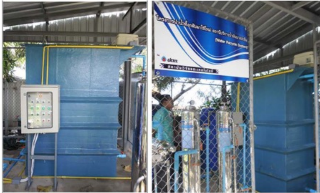
STAR" MBR Tank model OASIS-10 at PTT : Bang pa in Gasoline Station
