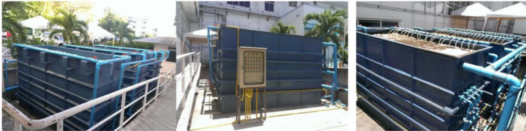
"STAR" MBR Tank model OASIS-150 at Samitivej Sriracha Hospital
