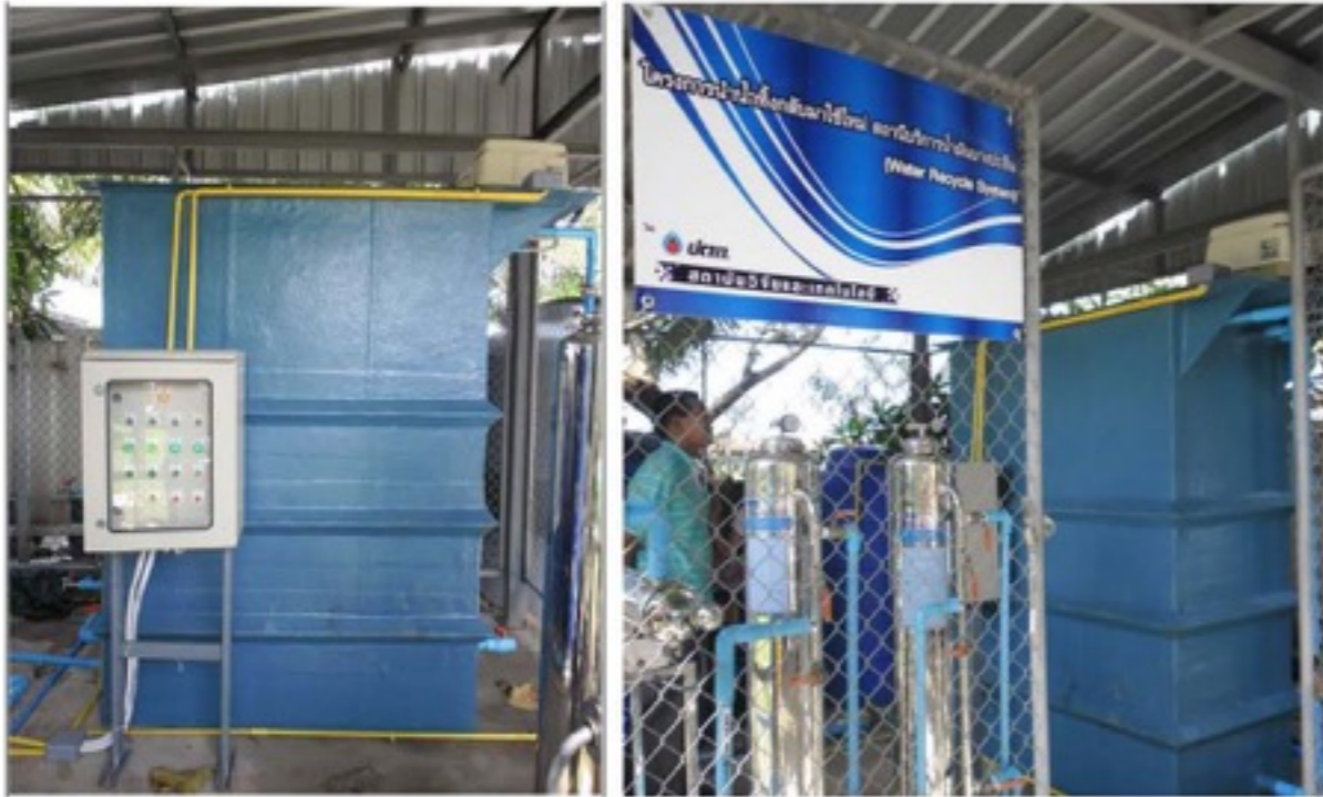
STAR" MBR Tank model OASIS-10 at PTT : Bang pa in Gasoline Station
